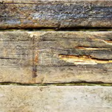
FACADE upper part
