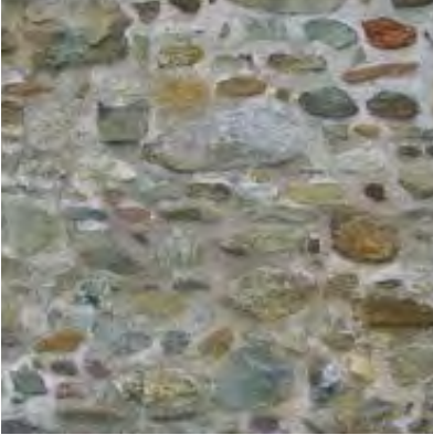
FACADE lower part
